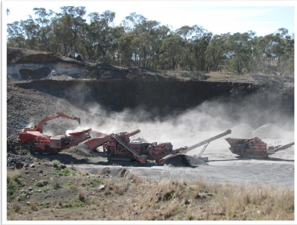
Production of aggregates and road base products underway at Warrumbungle Quarry
