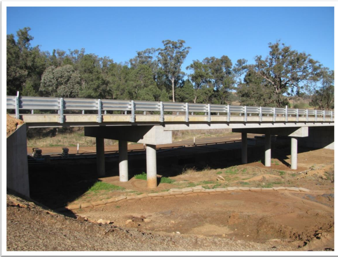
New bridge over Saltwater Creek No2 on the Purlewaugh Road
